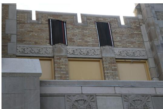
Black temporary protective screens are in place along the top of Twin Towers Middle School to capture crumbling cast stone masonry.
