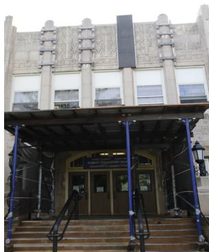
Twin Towers auditorium entrance has a black protective entry canopy, with reinforced masonry above. This captures crumbling cast stone masonry.
