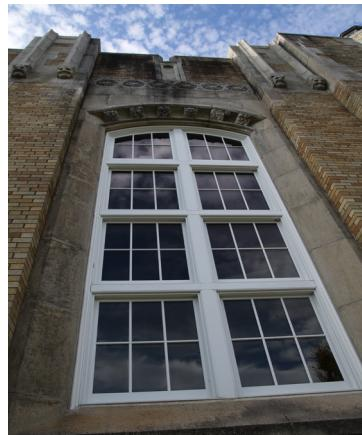
A typical Twin Towers auditorium window area, which requires masonry restoration and cleaning.
