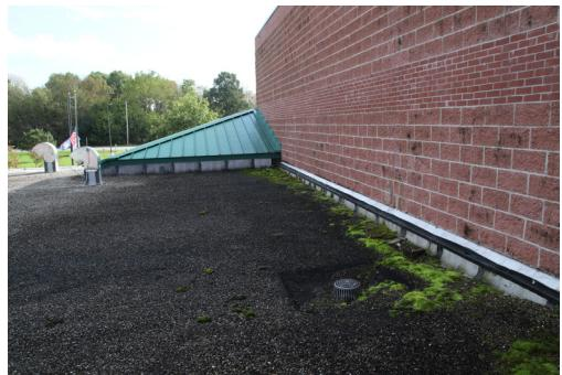
Monhagen Middle School roof has deteriorated and the masonry wall has significant water penetration.
