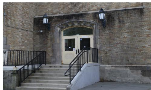
The side entry door area at Twin Towers Middle School requires masonry restoration, pointing, clearing and door/frame replacement.
