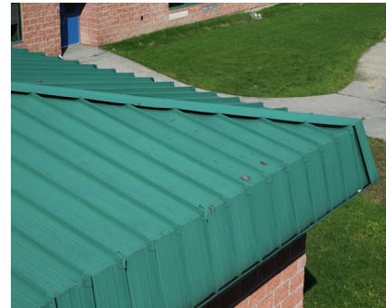
Maple Hill has failed roof detail with rusting through started on many panels.
